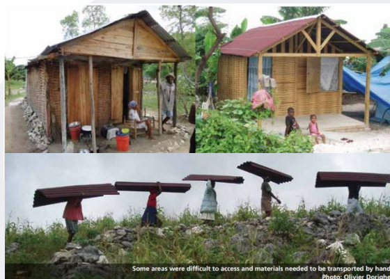
Some areas were difficult to access and materials needed to be transported by hand. Photo: Olivier Dorighel
